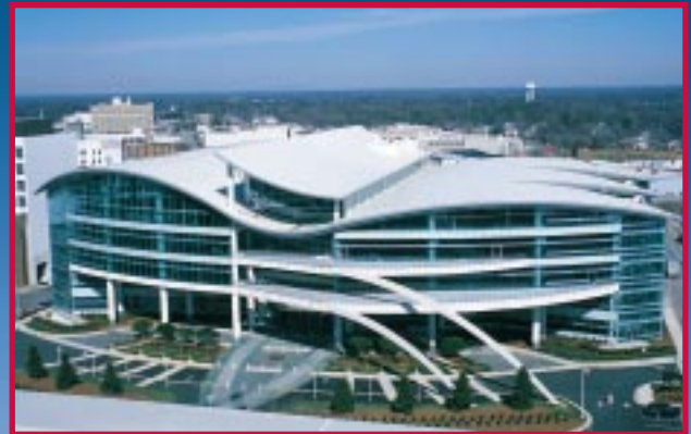
Showplace, High Point, North Carolina
